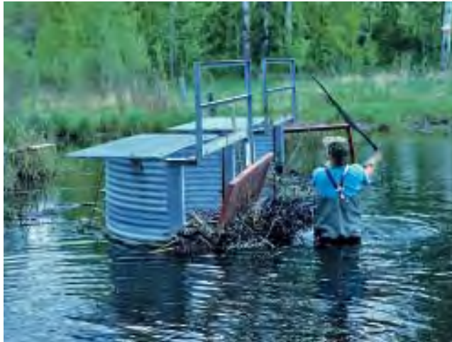
Cleaning a water control structure
