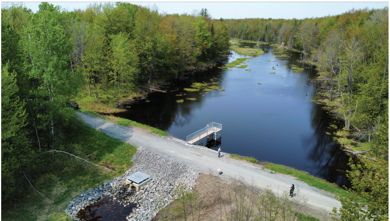
The Drummondville Restoration Project in Québec involved rebuilding a dike and water-control structure on 17.8-hectares (44 acres) of critically important wetland habitat owned and managed by the City of Drummondville/Ducks Unlimited Canada
